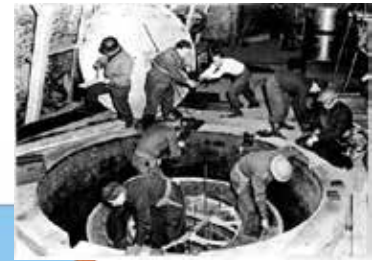
FIGURE 1: (top) the B-VIII reactor being disassembled by US and British personnel in 1945, (bottom) a cross section of the assembled reactor: an array of U-nat metal cubes suspended in heavy water, surrounded by a graphite reflector
