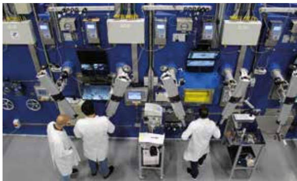
MRF staff operating manipulators in the hot cells © UKAEA
