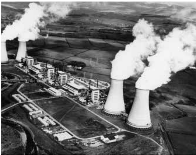
FIGURE 1: The four units of Calder Hall in operation
