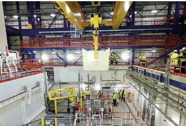
Figure 4. Test storage box successfully being lowered into the vault
