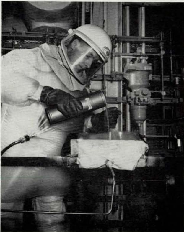
8—Pouring liquid nitrogen for partial freeze plug wearing protective clothing
