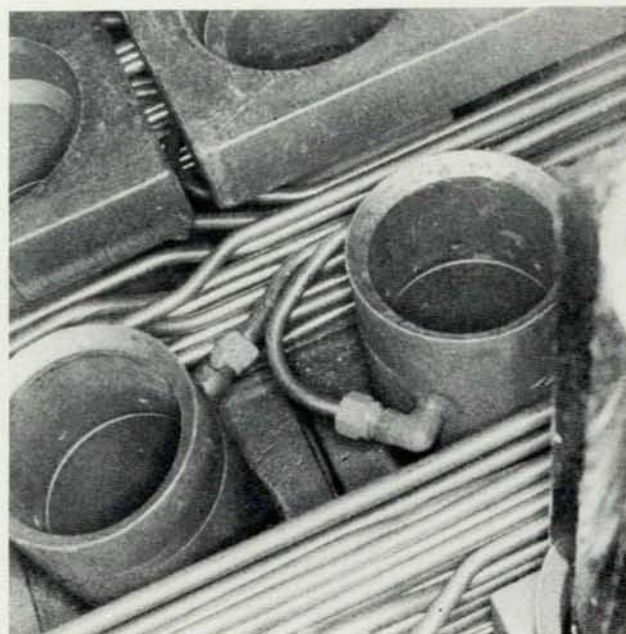
Fig 15 Trawsfynydd charge pan and charge pots
